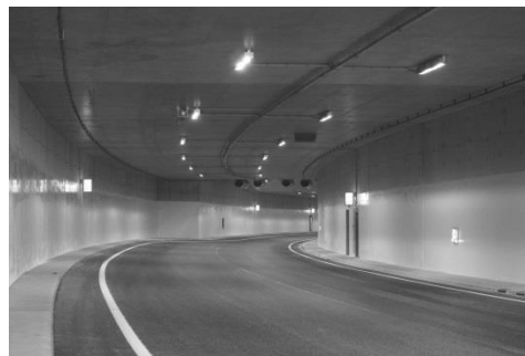
Picture 1: Tunnel entrance
