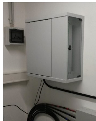
19" AP Sensing DTS device mounted in a flat wall cabinet
