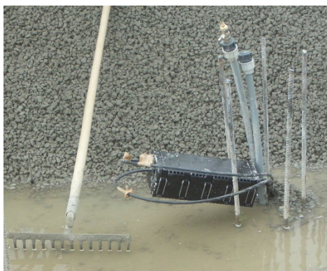
Joint box used to connect cables during installation
