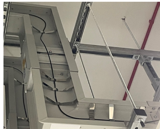
Above: Thermal image of cable installed along bus duct Below: Sensor cable fitted on bus duct
