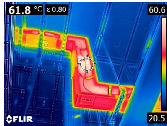
Above: Thermal image of cable installed along bus duct Below: Sensor cable fitted on bus duct
