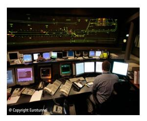
Four SAFE stations - around 900 meters long - will be equipped with AP Sensing linear heat detection and monitoring systems. Once a train has stopped at a SAFE station, the systems detect the exact location of any fire regardless of high air currents. The specific fire location data is used to trigger the Fogtec high pressure water mist suppression system with pinpoint accuracy.
