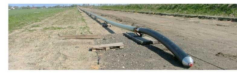
The sensor cable itself was pulled through five HDD sections, therefore a highly robust sensor cable was selected with double-armored protection. This not only ensured a safe installation, but also continuous operation in case the pipeline rolls or shifts, which can alter the cable's position e.g., from the top to the bottom of the pipeline.
