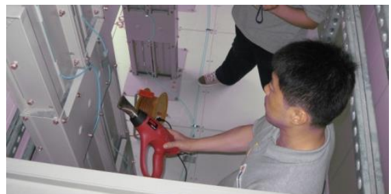
Commissioning and testing phase
