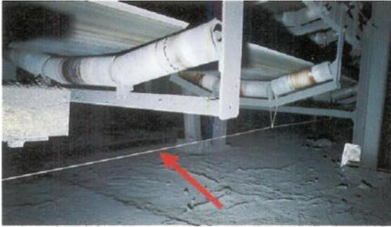
Figure 2: Installation of a sensor cable for detecting smouldering fires
