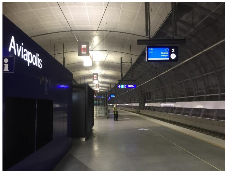
Aviapolis metro station is now monitored by AP Sensing
