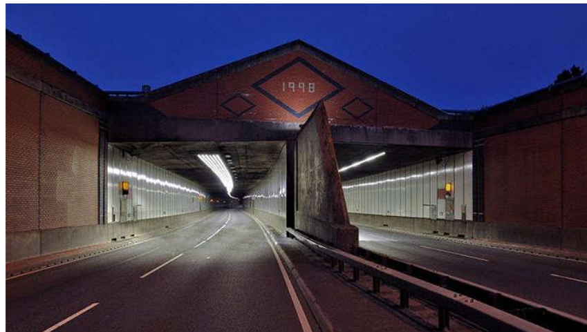
The Meir tunnel, ready for overnight testing
