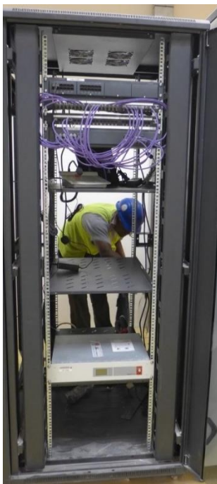
19" rack mounted Linear Heat Series during installation
