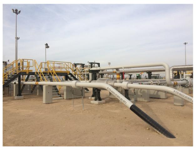
CO<sub>2</sub> pipeline exits the receiving station and proceeds 2 m underground
