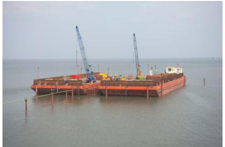
Floating excavation platform
