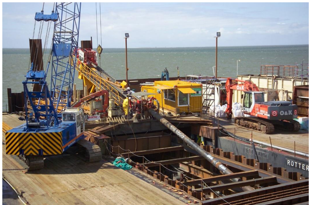
Laying the pipeline including sensor cable
