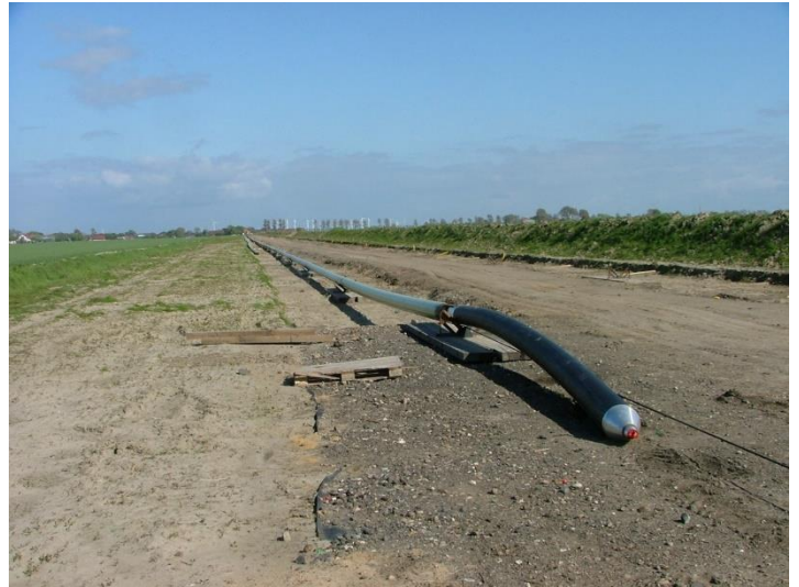
Pulling knob for pipeline installation including sensor cable
