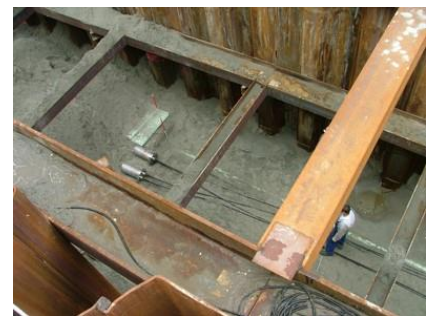
Joints for the mud flats, also shown in their construction trenches
