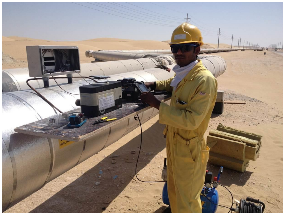
Splicing and installing fiber optic sensor cable
