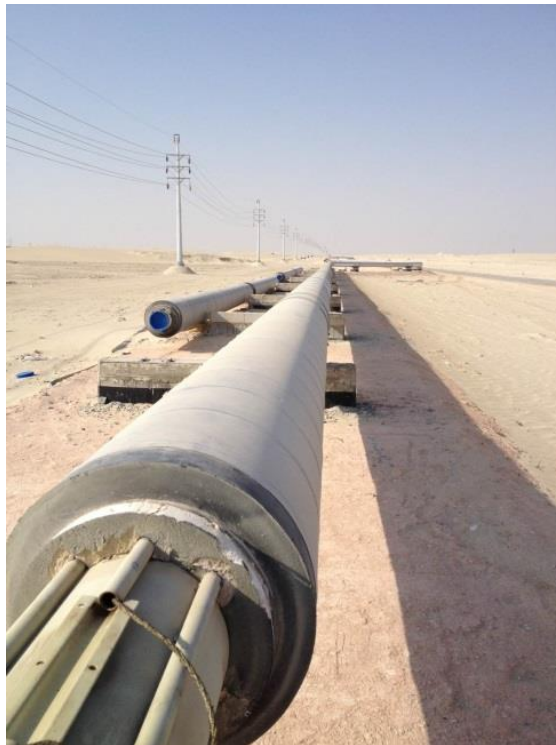
Sensor cable installed between the pipe and insulation
