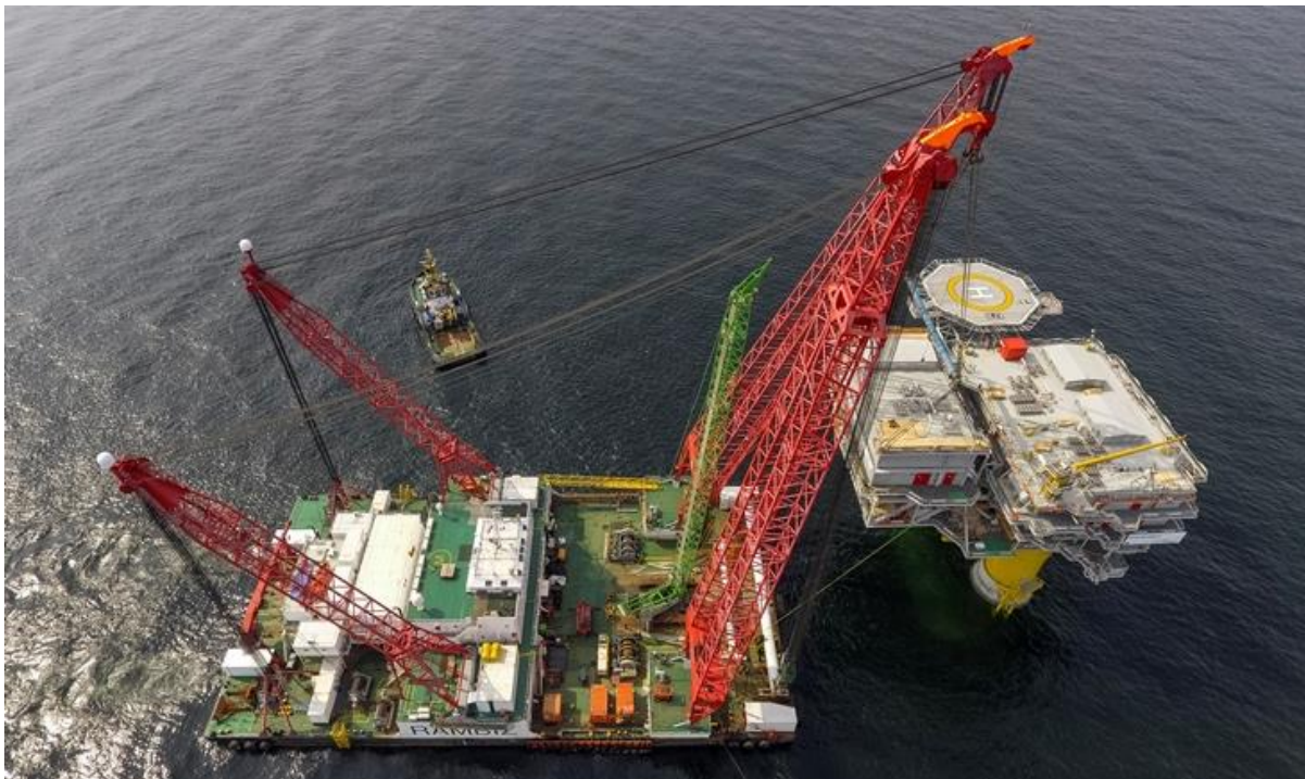
Kriegers Flak platform installation ©Energinet
