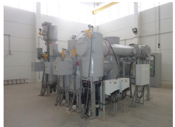
Trefoil configuration in the substation; the GIS switching room
