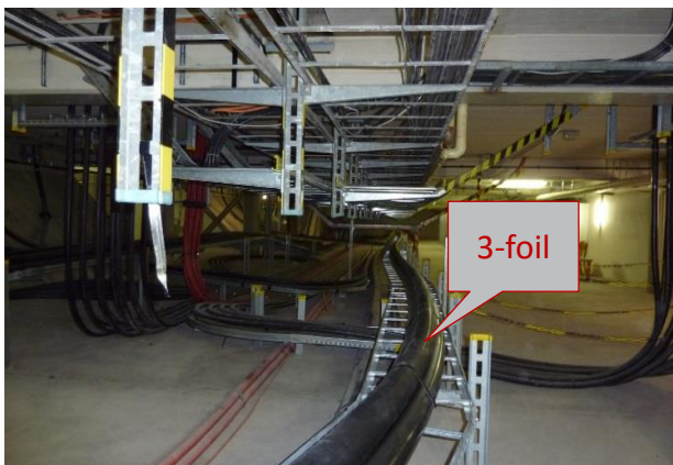
Trefoil configuration in the substation; the GIS switching room
