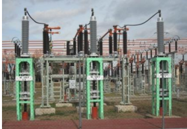
Cable starting point
