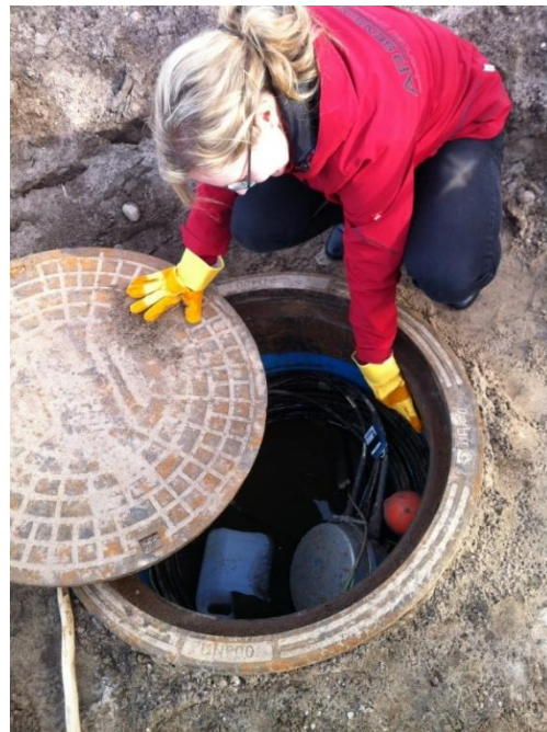
Installation of the DTS system at the Lithuanian site
