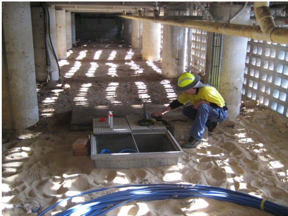
Sensor cables being prepared in the substation
