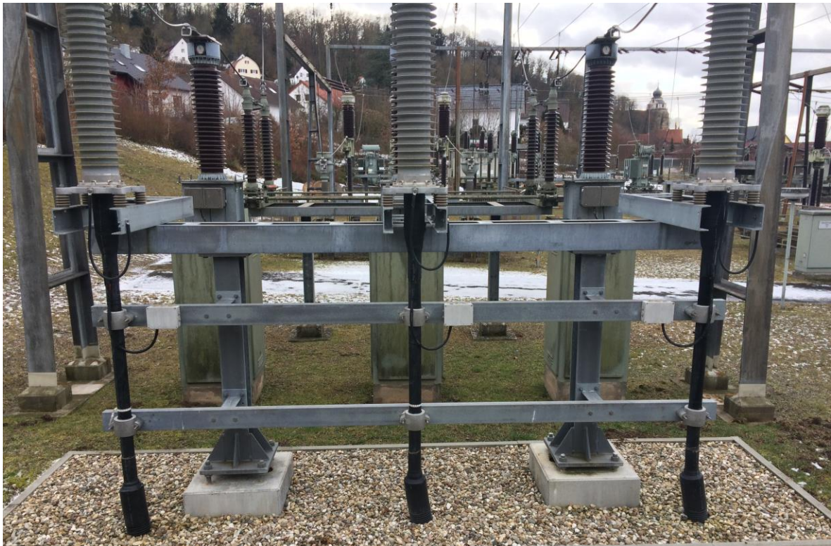
Power cable in Herrenberg substation
