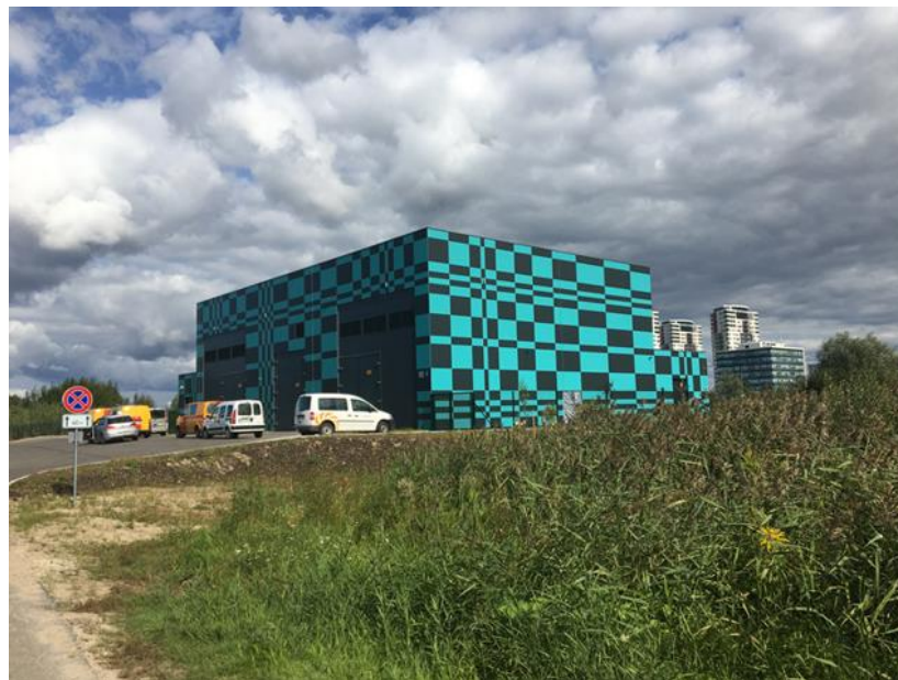
New substation in Riga
