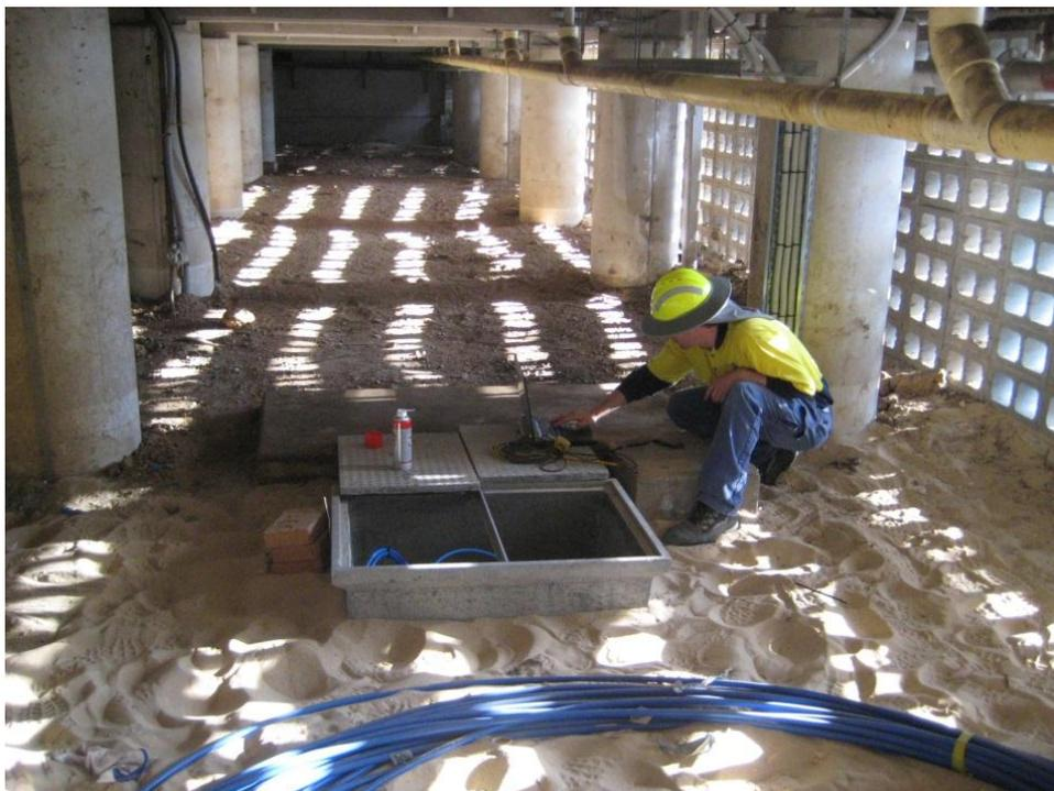
*Sensor cables being prepared in the substation*
