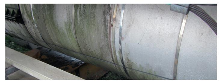
Fiber optic cable installed along terminal pipe
