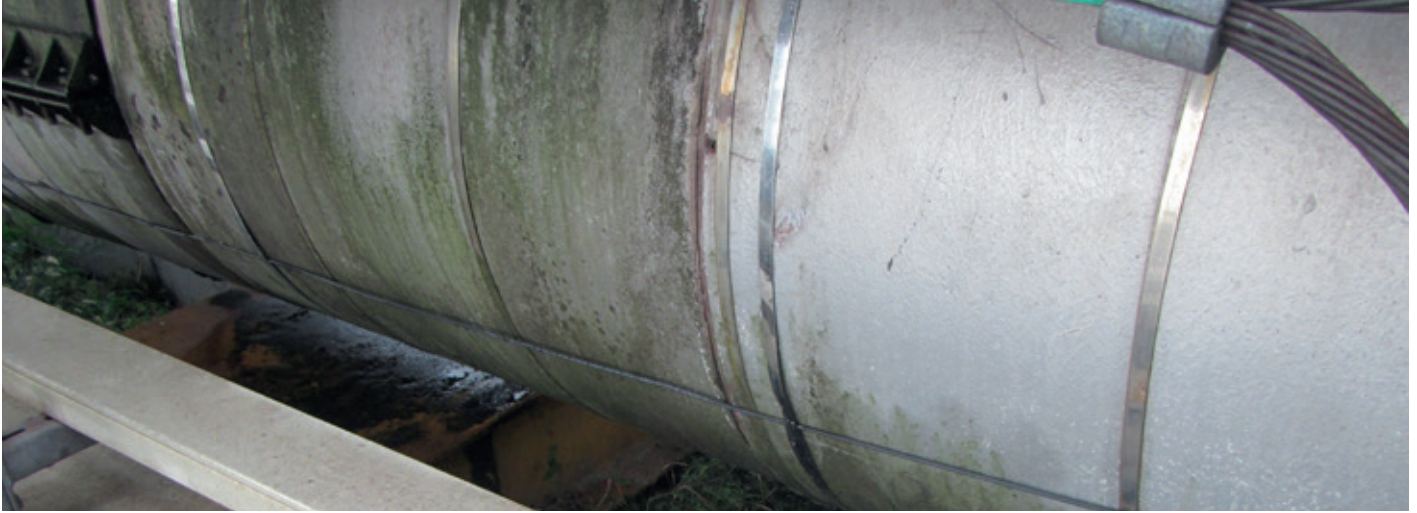
Fiber optic cable installed along terminal pipe
