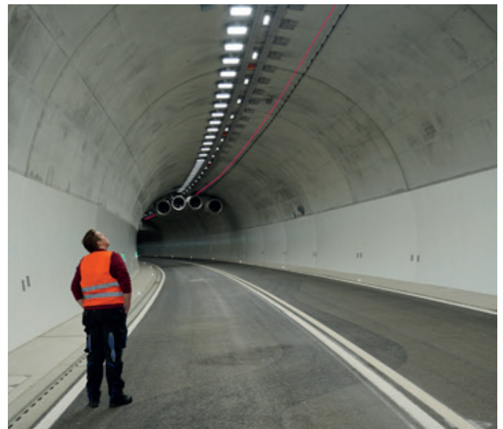
Figure 2: Fiber optic cables, highlighted in red for visibility
