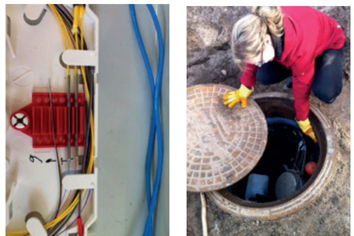
Figure 2: Power Installation of the DTS system at the Lithuanian site
