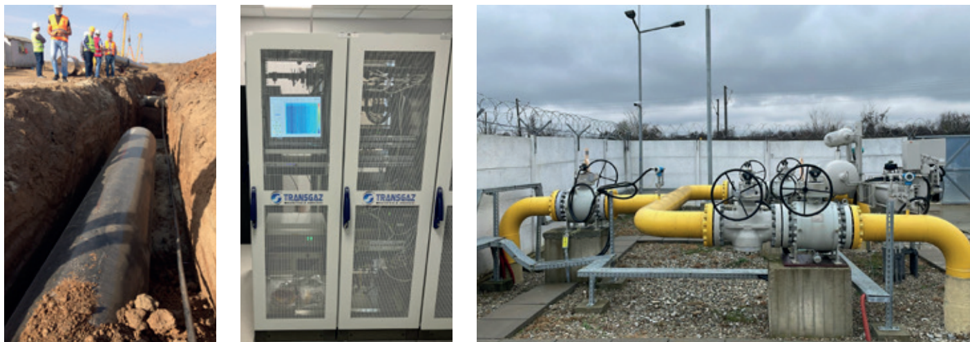
Figure 1: BRUA pipeline with FOC duct during the installation phase and monitoring cabinet located in one of the valve stations
