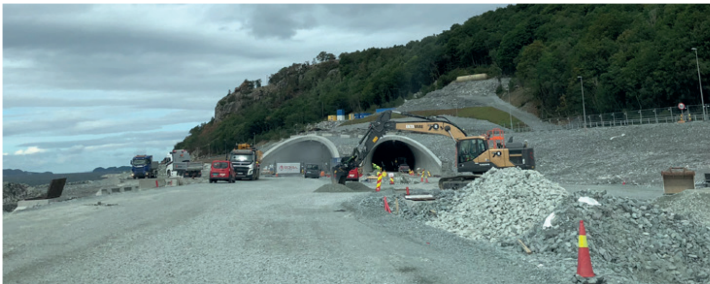
Figure 1: Construction of the Ryfast Tunnel System
